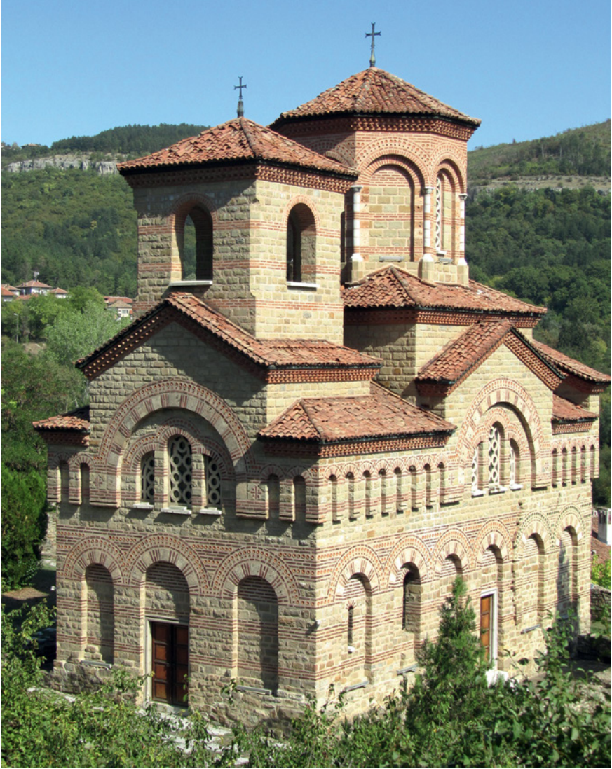
FIGURE 1 The Church of Saint Demetrios in Tărnovo, as now rebuilt. AUTHOR'S PHOTO.
